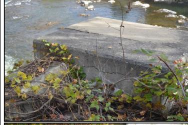
Top of Left Abutment showing cracking
