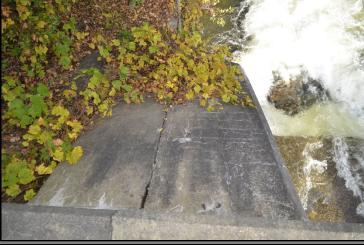
DS Side of Left Abutment showing vertical Crack
